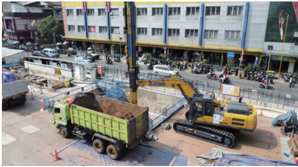
Jakarta MRT Project Several XCMG XEG2600 telescopic excavators were contributing to the construction of the second phase of the Jakarta MRT North–South Line project. Serving as pioneers in this infrastructure endeavor, they were tasked with the critical role of initial earth excavation.
