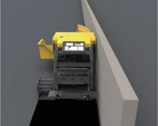
Construction against the wall
